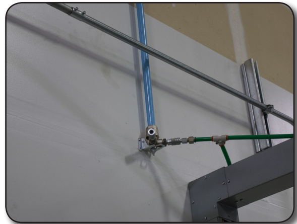
FIGURE 2. CENTRAL AIR DELIVERY QUICK RELEASE VALVE
